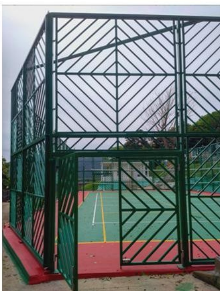
The campus volleyball court fencing and entrance after the renovation
