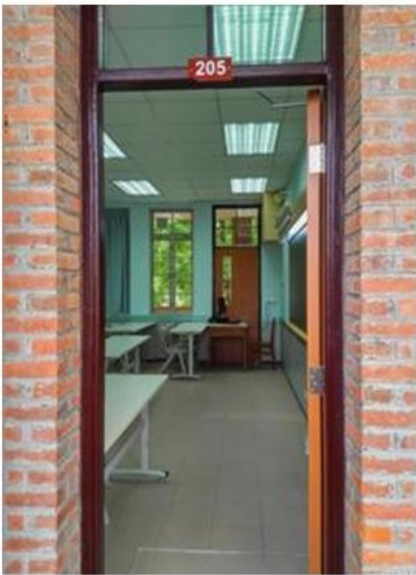
Peering into the newly renovated classroom 205 with its ceiling lights switched on
