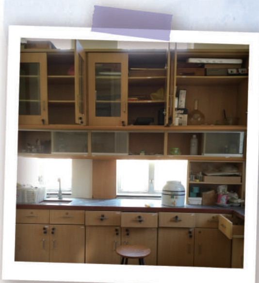
Former Chemistry Lab built-in cabinets, sink, and lab stool seat in the smaller, adjoining room
