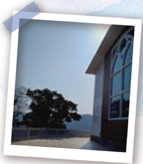
New back walkway and new granite railing
