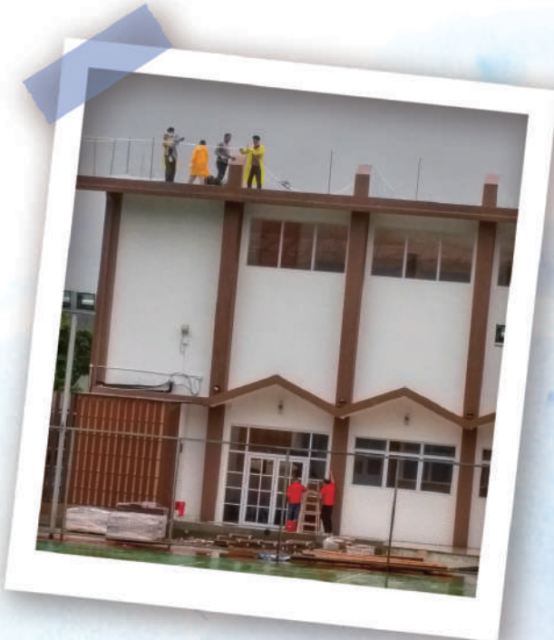
Exterior renovations occur at King Huy Hall
