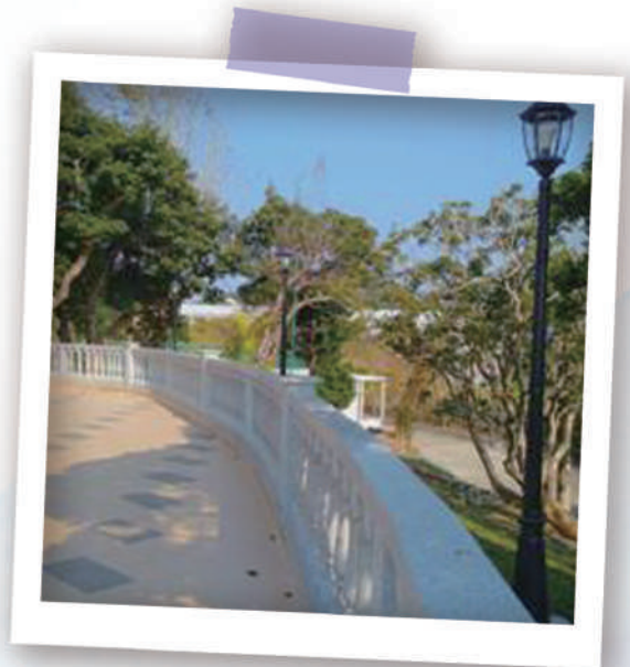
New side walkway and granite railing
