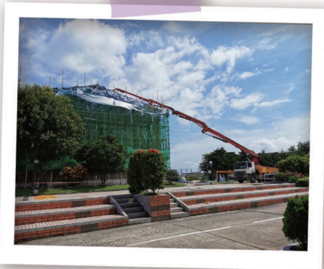
Forklift helps with HKAC Admin. Building rooftop waterproofing and repairs projects
