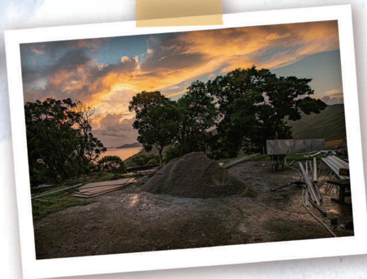
Dawn breaks during the second renovation phase, which included the back part of Bayview Church / King Huy Hall.
