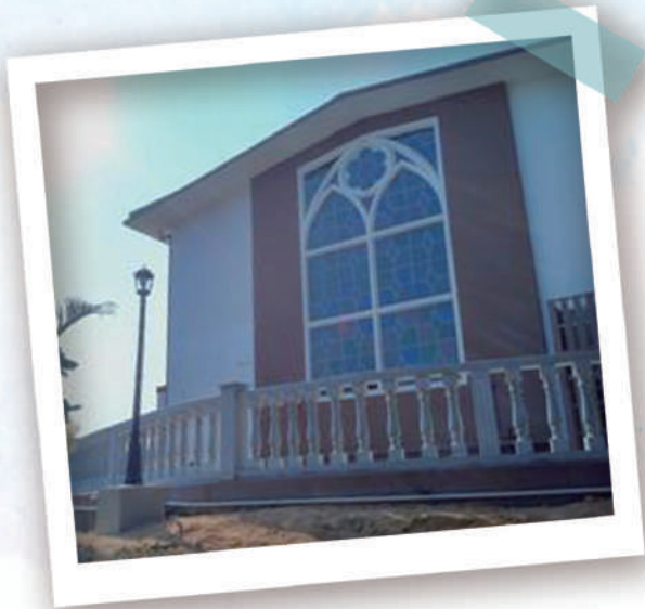
King Huy Hall with new waterproof roof
