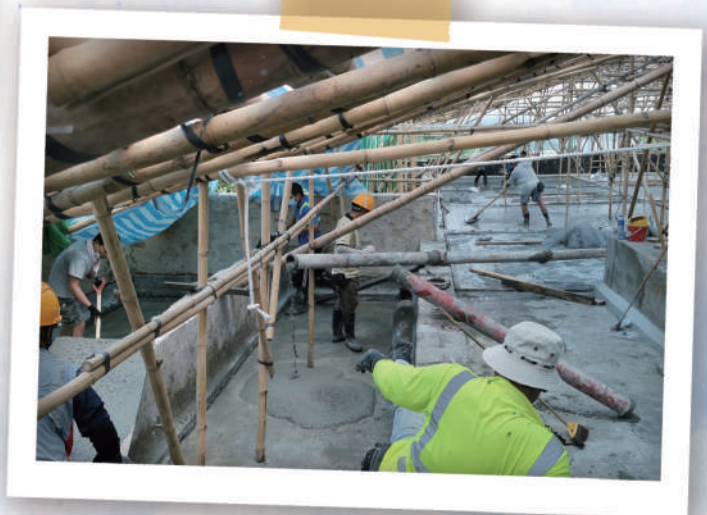
Above and below: Waterproofing work on the HKAC Admin. building rooftop
