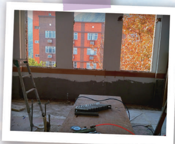
Rewiring work in Biology Lab classroom and a dormitories view
