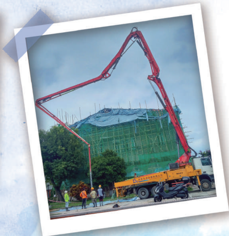
A forklift elongates to help workmen
