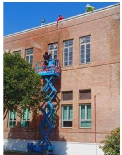
Lowering a water hose to allow the spraying down of bricks outside the Biology Lab classroom
