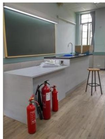
Fire extinguishers near the teacher's desk, green chalkboard, lab stool seat, corner window
