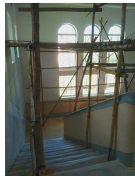
Stairwell heading down to the ground floor
