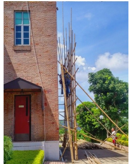
Workmen assembling the bamboo scaffold on the side of the Marketing team office
