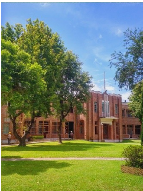
A sunny summer day in July 2020 with the scaffold about to be erected on the HKAC Administration building
