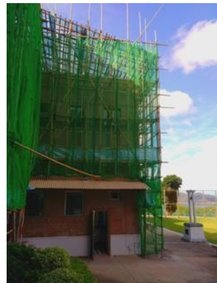
Back facade view towards the bell tower
