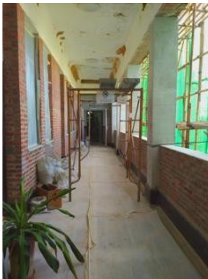
Second floor renovation view
