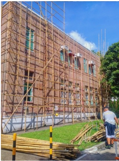
One side of the HKAC building
