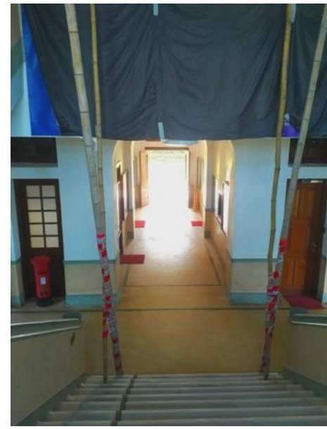
Peering down the interior stairwell
