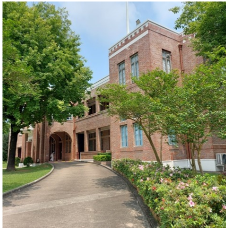
The beautiful, 84 years old, grade 2 historic HKAC Administration Building in springtime
